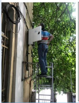
It has a built-in heated input to reduce the influence of humidity on the measurement of dust particles. Wireless and cellular data transfer for remote access. Possibility for WIFI tool network.
